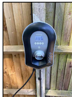
Zappi multiphase, car chargers With selectable power settings of 7kW and 22kW,
