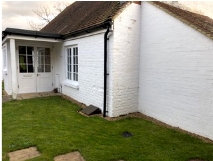
Figure 6 - View towards front of 7 Dairy Farm Lane from approximate position of 8 Dairy Farm Lane Study window
