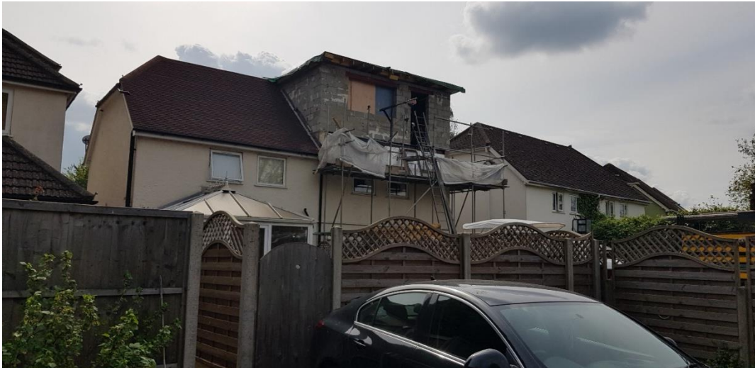
Rear view of nos. 1 & 2 Maygoods View
