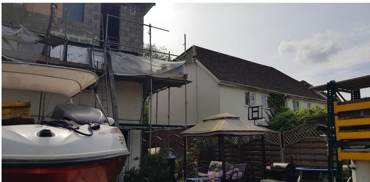
Looking towards the rear of no. 3 Maygoods View.
