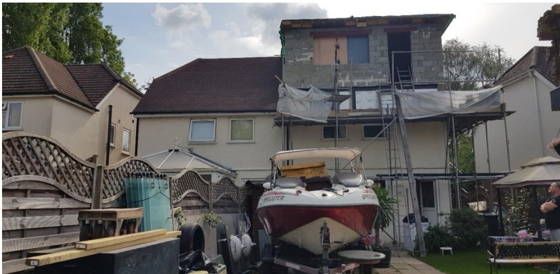
Rear view of nos. 1 & 2 Maygoods View
