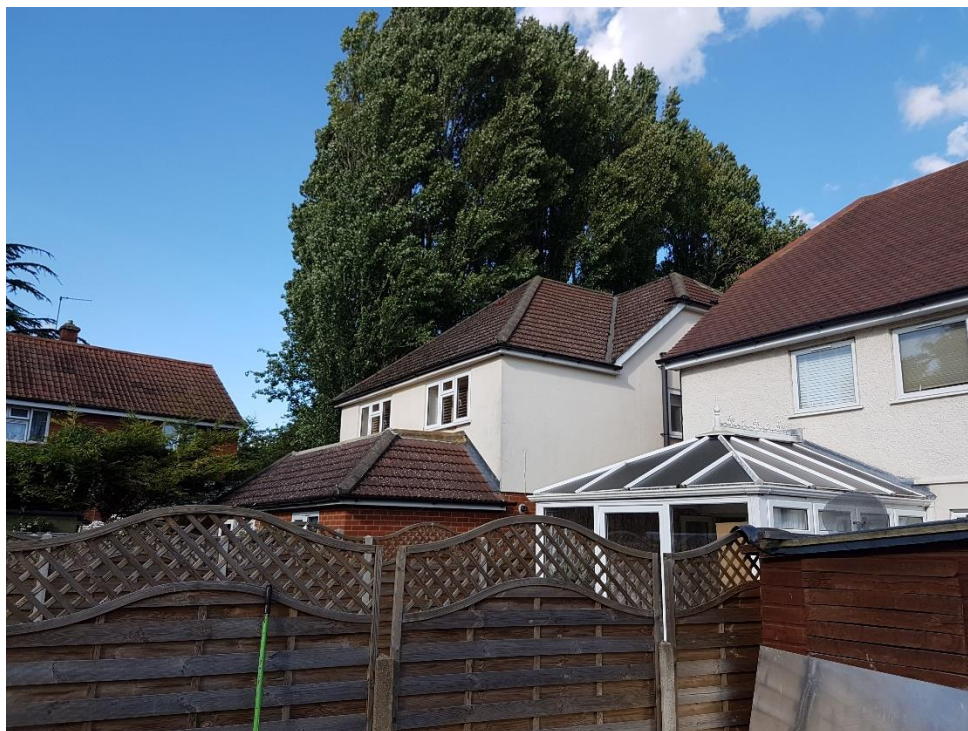
Looking towards the rear of no. 1A-C Maygoods View.
