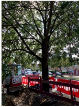
T1 Trenching works in progress. Many roots severed.
