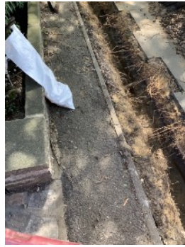
T1 Trenching works in progress. Many roots severed.
