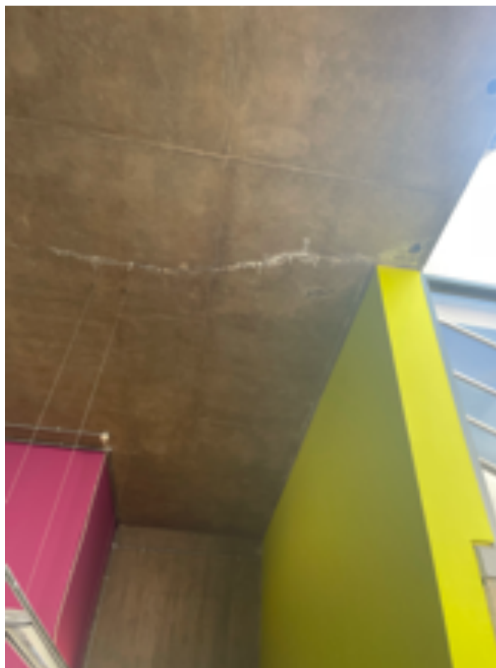
Fig.7 fine crack to concrete starting in corner directly below rooflight.
