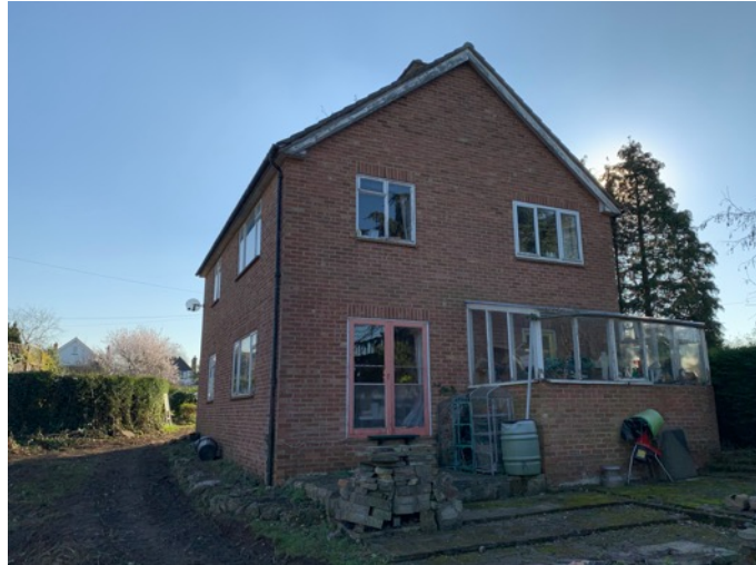
Photograph 9: Rear (north gable).
