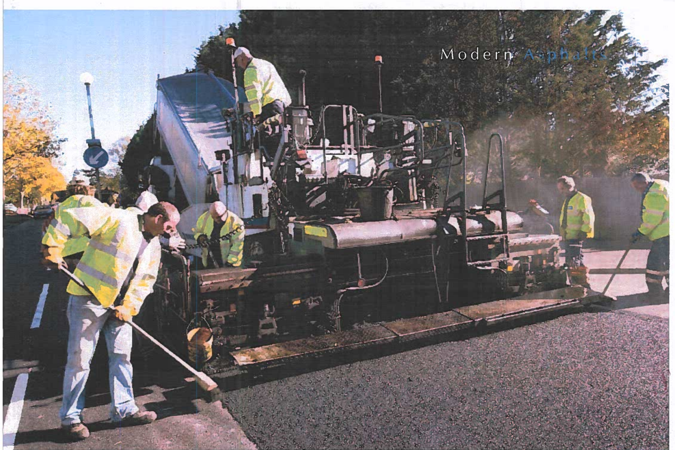
Ringway's 'Ultraphone' surfacing is laid on the A26 near Tonbridge in Kent to reduce noise the equivalent of a 75% reduction in traffic flow
