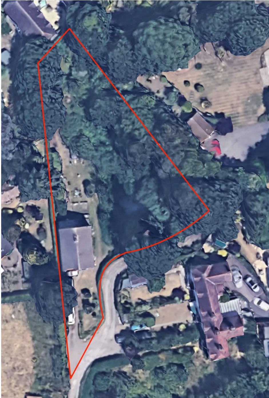
Figure 2: Aerial photograph of the site.
