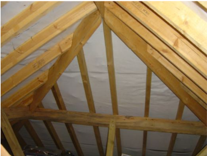
View of roof construction of the side extension
