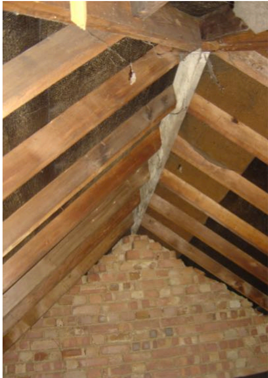
View of party wall between no. 3 and no. 5 and the original roof ridge
