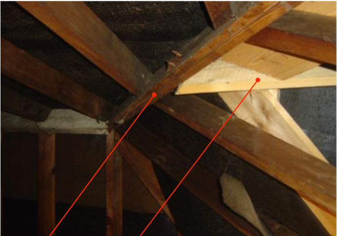
View of old ridge and extension ridge junction (looking up)
