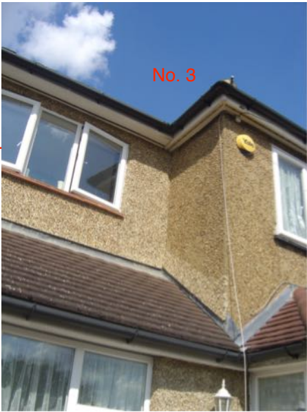
View of junction between roof of extension and front porch
