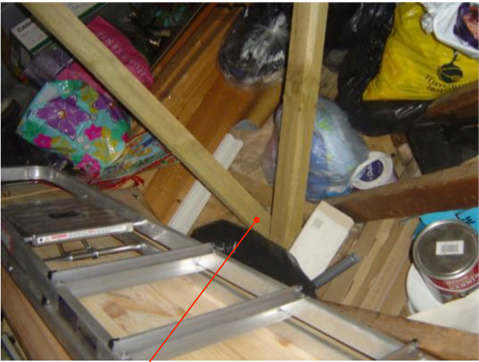
View of extension purlin props to side extension, as existing
