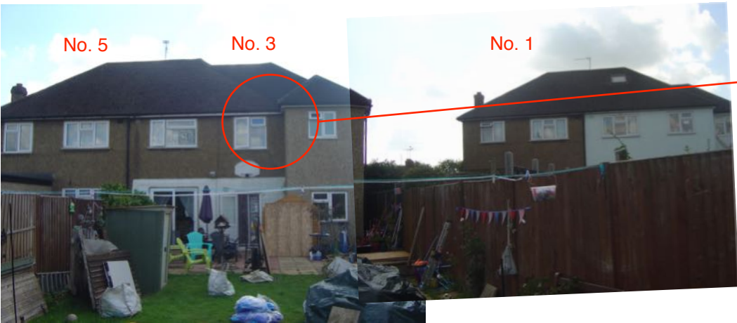
View of rear elevation
