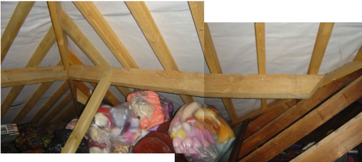
View of rear purlin and prop junction
