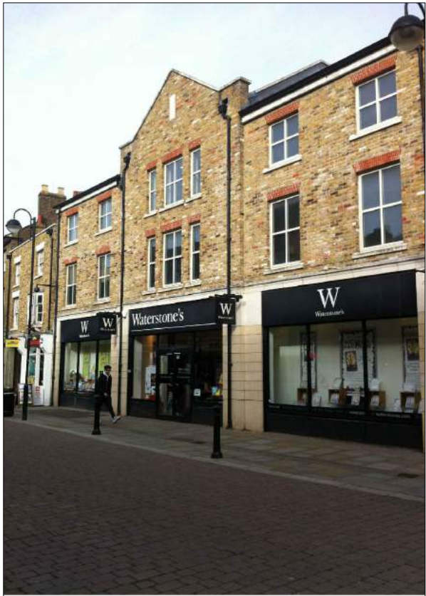
C EXISTING - PHOTO REF 01
