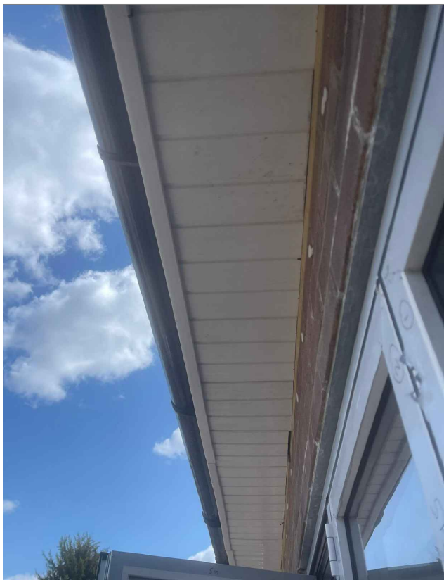
As Build photograph 03 Rear elevation the overhang of the roof contractions on the single storey rear extension is reduced to 20 centimeters.
