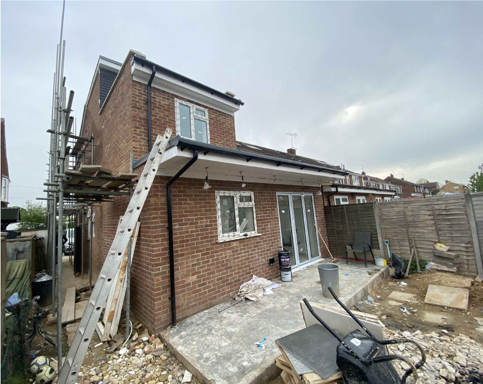
As Build photograph 01 Rear elevation construction of an overhang of the roof on the single storey rear extension 90 centimeters
