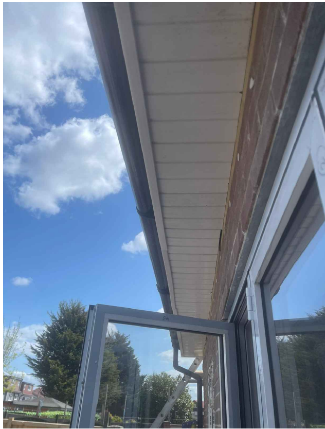
As Build photograph 01 Rear elevation construction of an overhang of the roof on the single storey rear extension 90 centimeters
