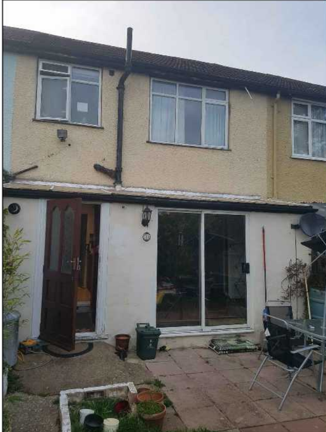
Rear elevation with existing 1.5m extension which will be replaced by proposal
