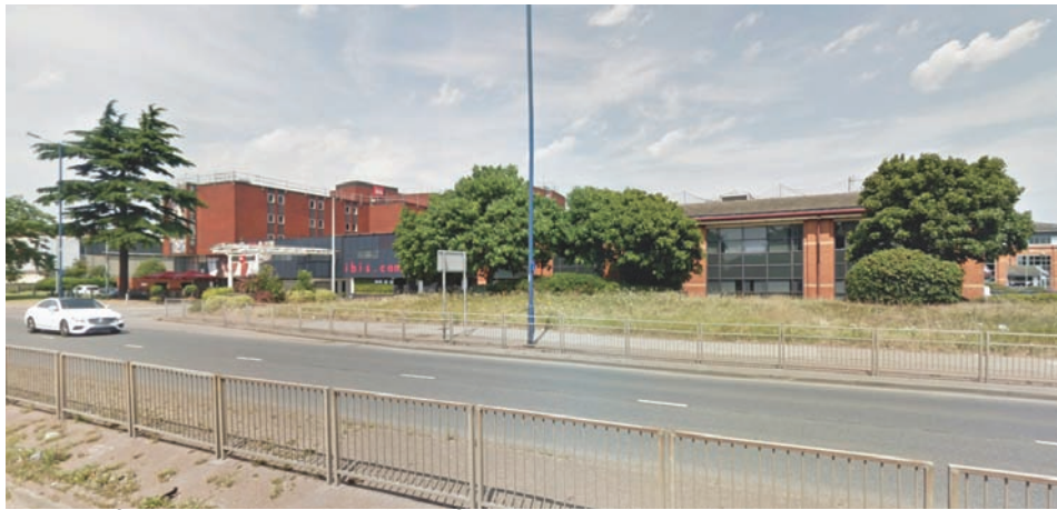
1. View of the Ibis hotel and Building 2 from Bath Road
