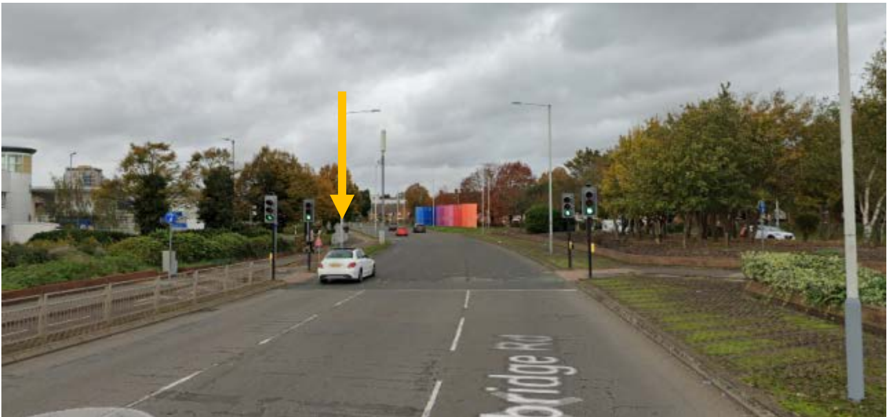
View of the existing equipment from roundabout exit
