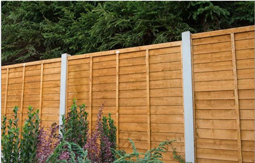
Timber fence panels with concrete posts
