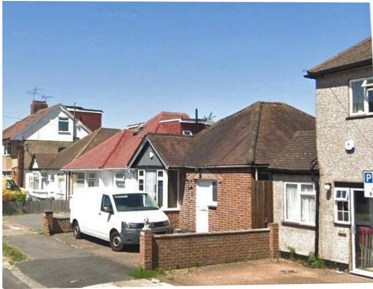
13 Mahlon Avenue as existing
