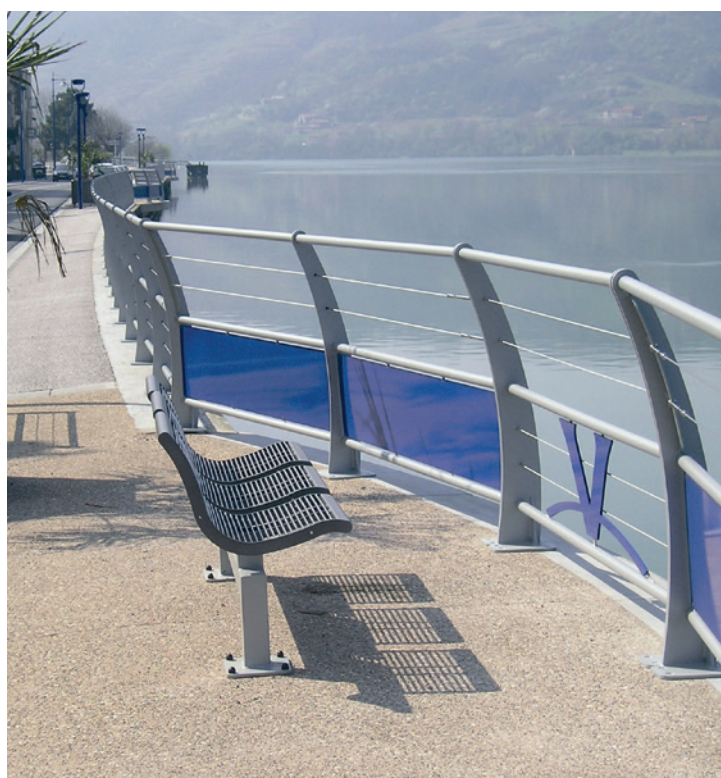
Series 9600 steel uprights with stainless steel cables with bespoke panels and Saint Vallier logo, Belvedere Saint Vallier.
