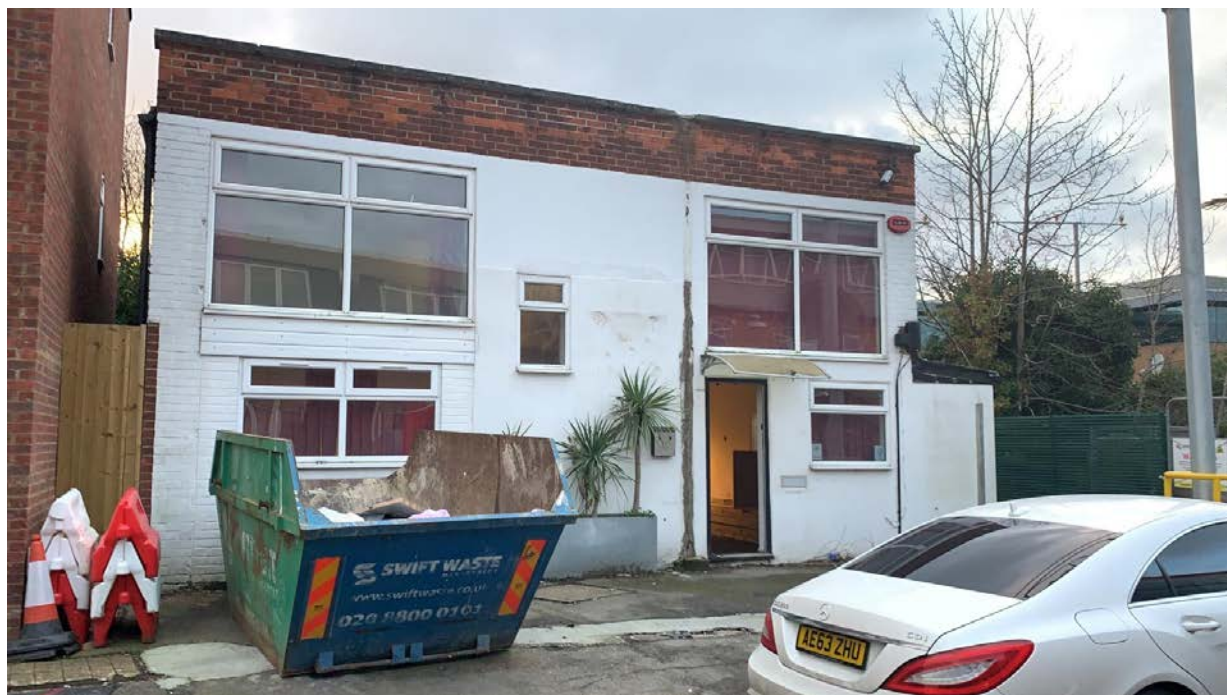
Photograph 1: View of front of the property.
