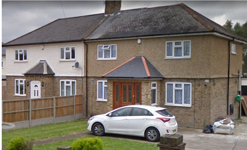
Figure 2: Existing front elevation (Google images). This shows a single outfall pipe serves the pair of semi-detached dwellings.
