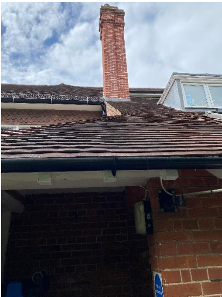
Picture 11: Example of a couple of loose tiles on the eastern elevation of B1.
