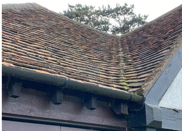
Picture 25: Example of loose tiles on the roof of B3.
