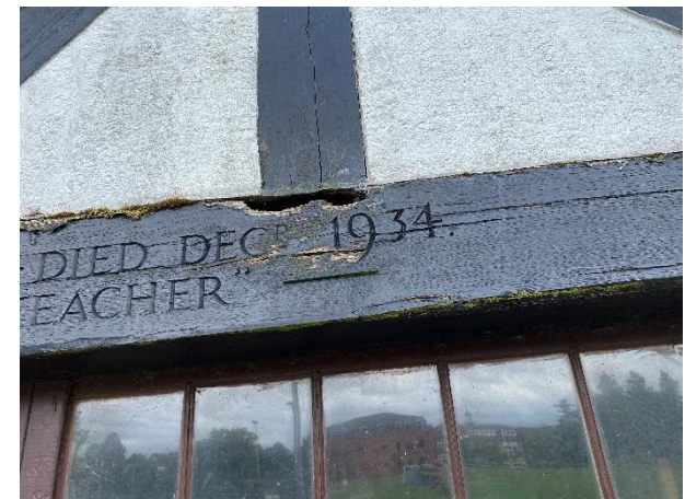
Picture 26: Hole leading into in the B3 on the northern elevation.
