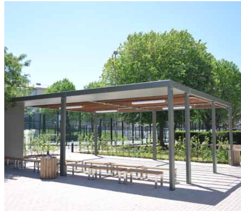
Canopy structure installed at Clapton Girls School, Hackney
