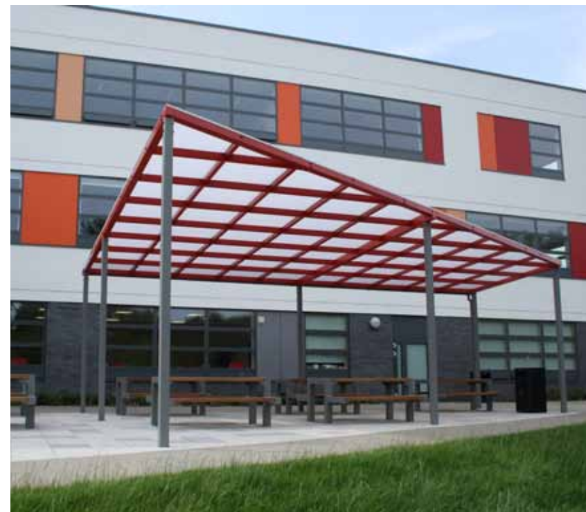
Canopy structure installed at Oasis Academy, Mayfield
