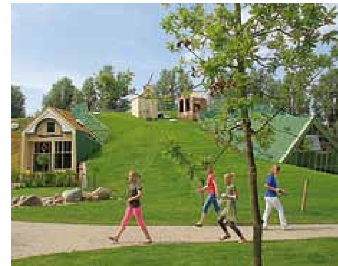
Steep gradient green roof treatment
