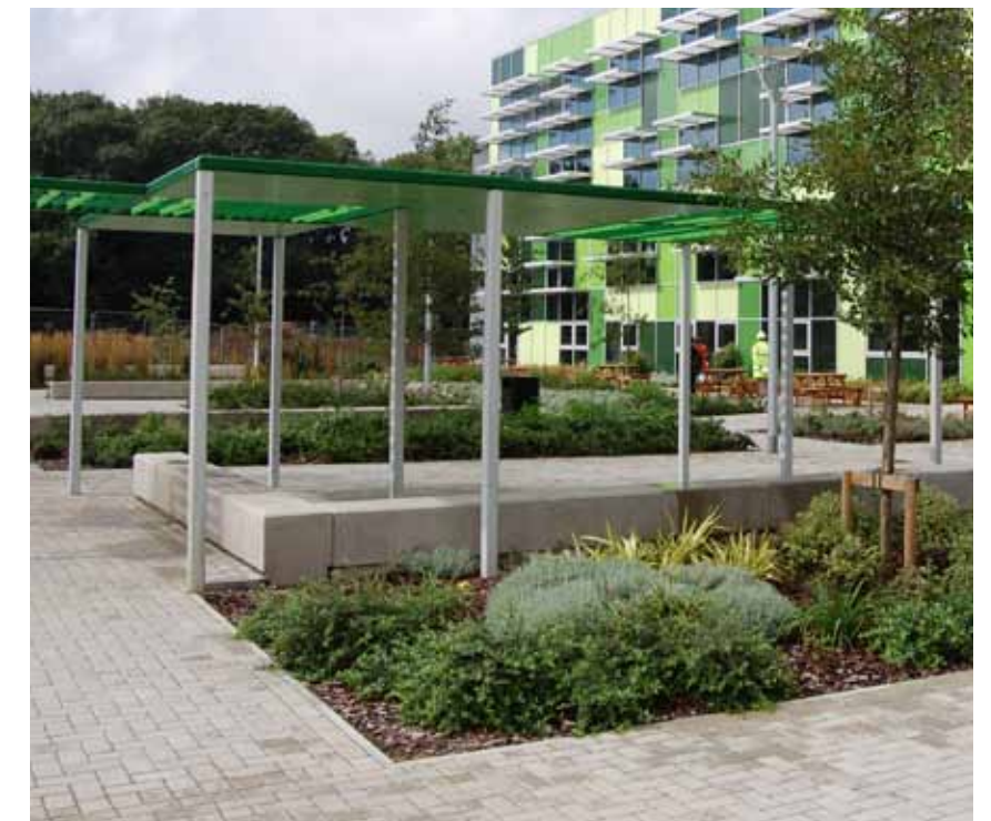
Canopy structure installed at New Line Academy, Maidstone
