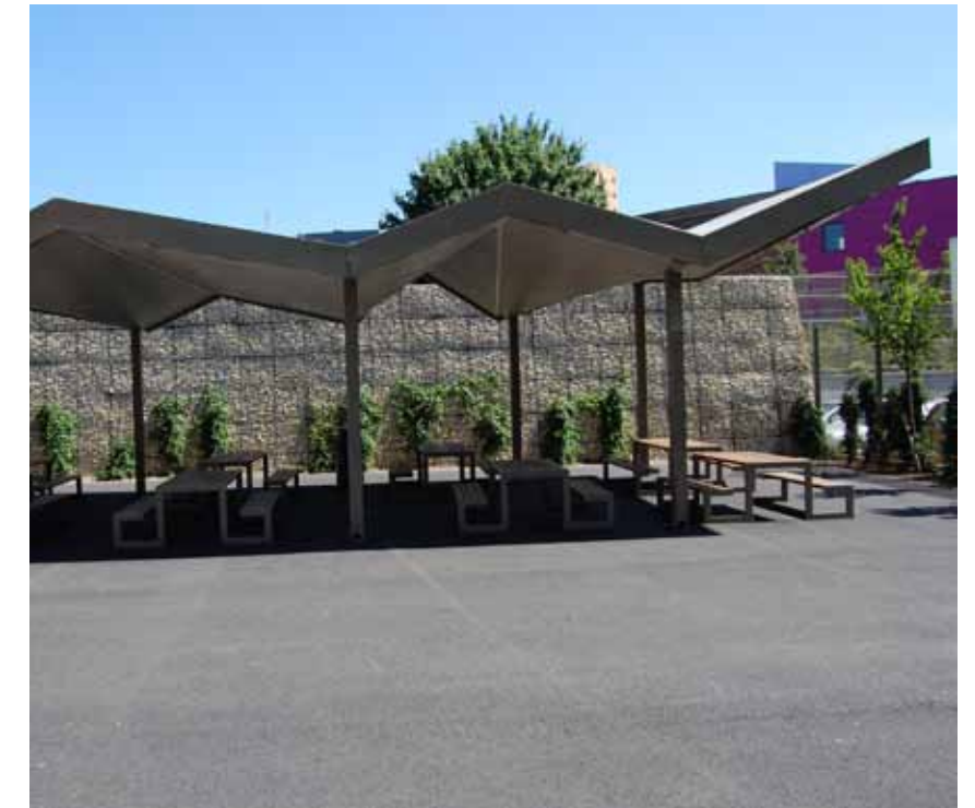
Canopy structure installed at Cardinal Pole, Hackney
