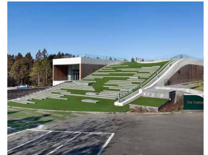
Intensive green roof rising from ground level
