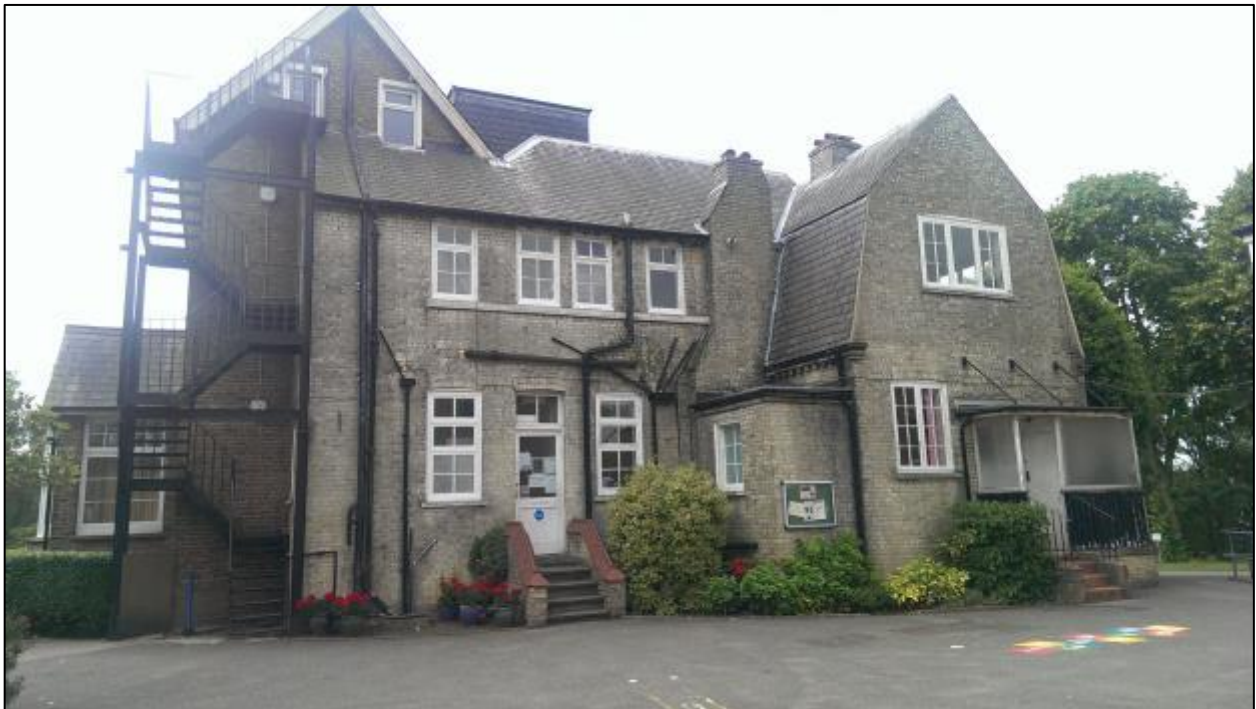
Figure 2: The Northern elevation of B1.
