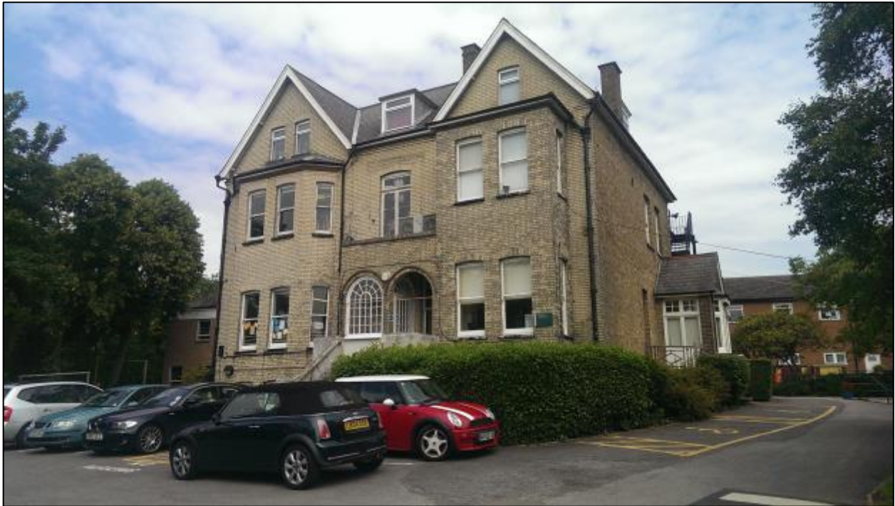
Figure 1: The Southern elevation of B1.
