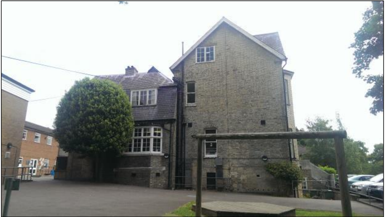
Figure 3: The Western end of B1.
