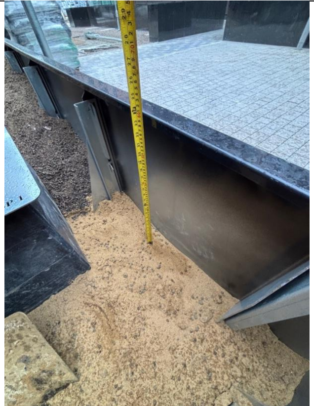
Thickness example (600mm) within podium prior to topsoil placement in Block F
