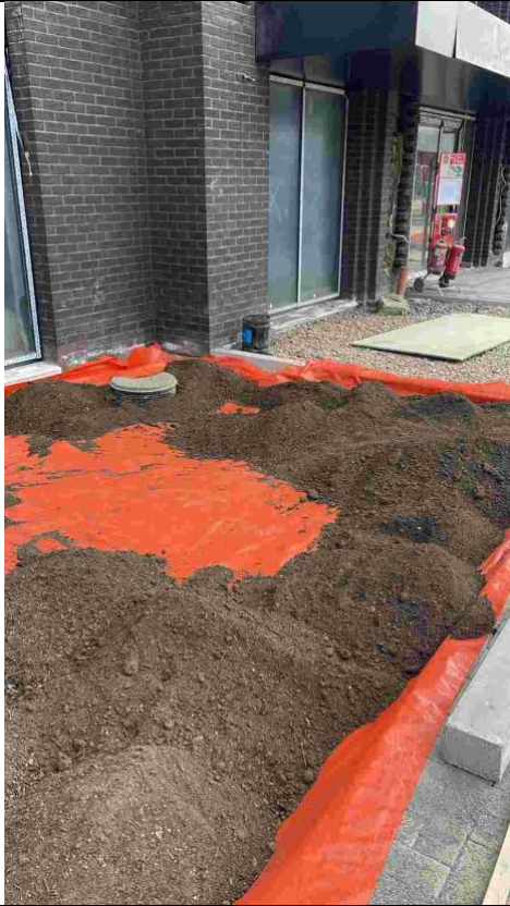
Representative photos showing marker layer and topsoil within area of installed utilities in Block F
