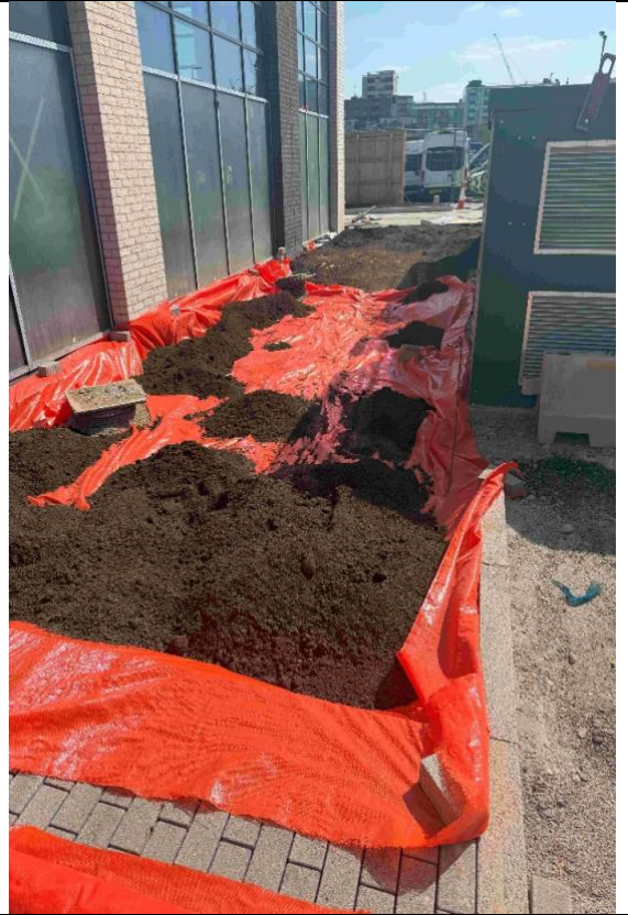
Representative photos showing marker layer and topsoil within area of installed utilities in Block F
