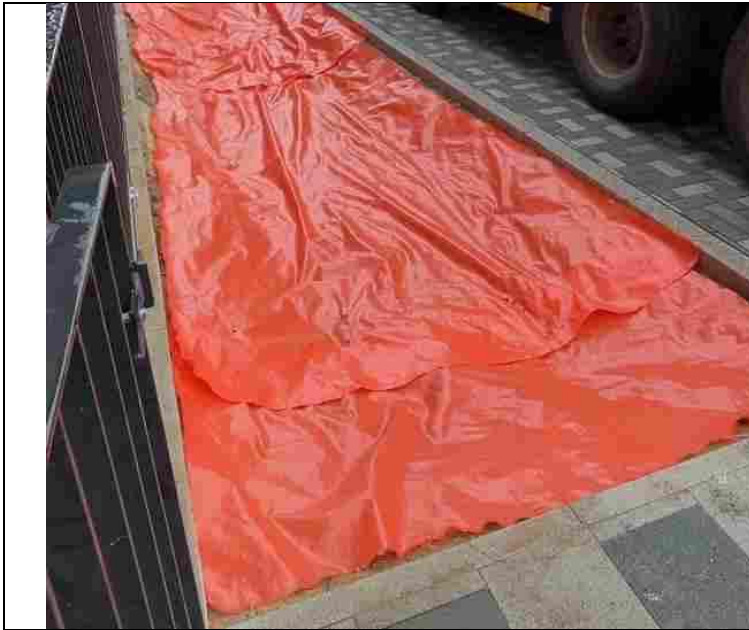
Example of marker layer laying and lapping with concrete (Blocks A and D)
