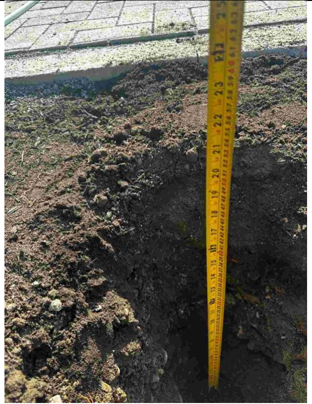
600mm thickness example within Block F (Ground Level)
