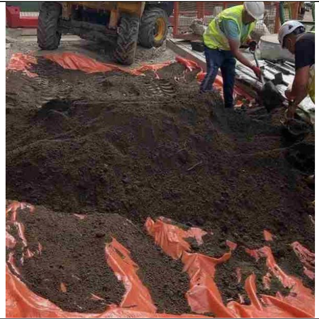
Example of marker layer laying and lapping with concrete (Blocks A and D)
