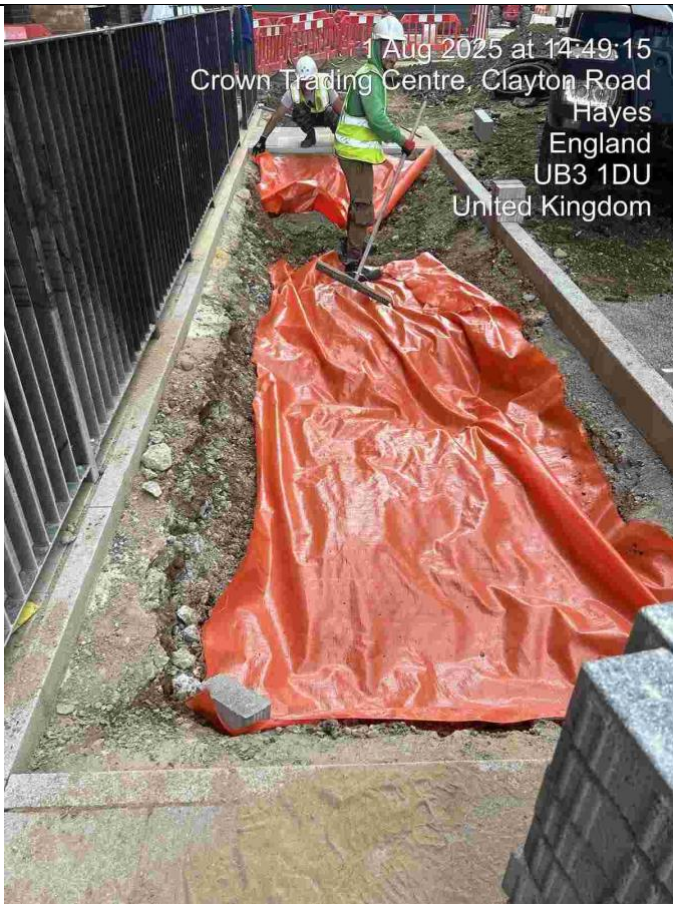
Example of marker layer laying and lapping with concrete (Block B)
