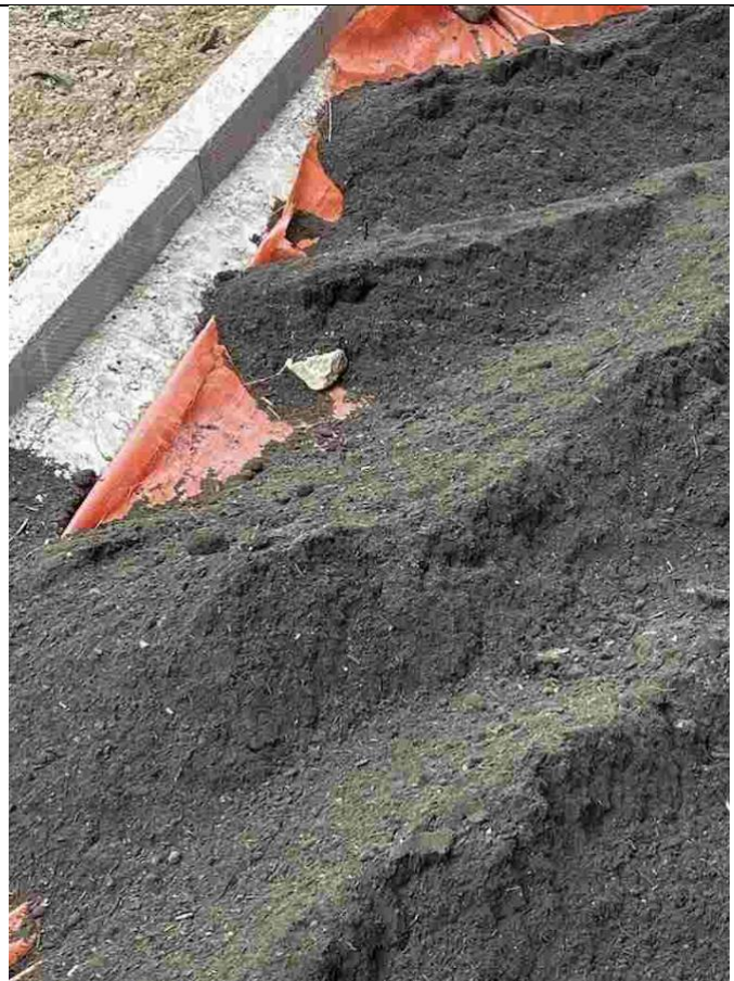
Example of marker layer laying and lapping with concrete (Block B)
