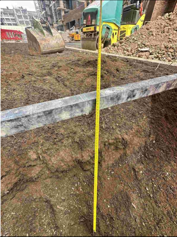
Example of 60cm topsoil thickness (Block B)
