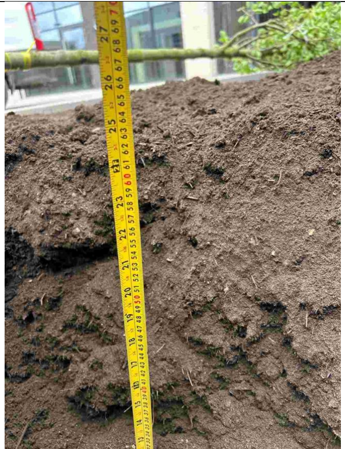
60cm Depth of Topsoil (Block C – Example)
