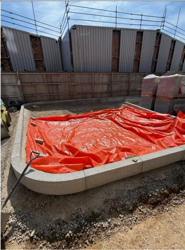
Marker Layer being laid (Block C – Example)
