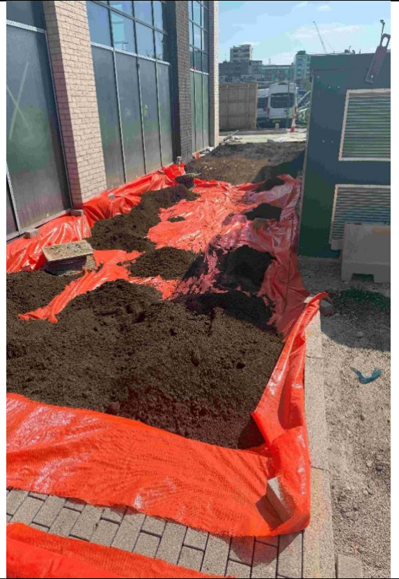
Representative photos showing marker layer and topsoil within area of installed utilities in Block F
