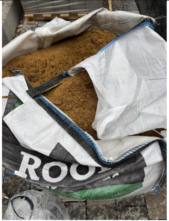
Representative photo showing bulk bag with imported sand prior to placement (laid under the 600mm of topsoil at podium level)
