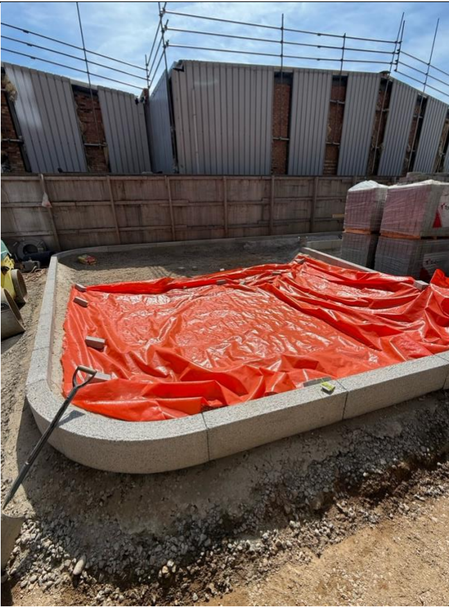
Marker Layer being laid (Block C – Example)
