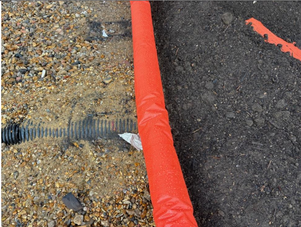
Representative photo showing marker layer and topsoil within asset protection in Block F
