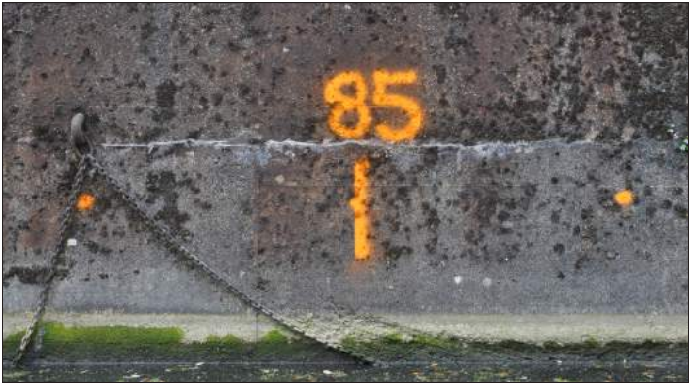
Fig.40 85m chainage - Debris steel tubing - on bed 10mm sticking out plinth along wall at base all satisfactory.
