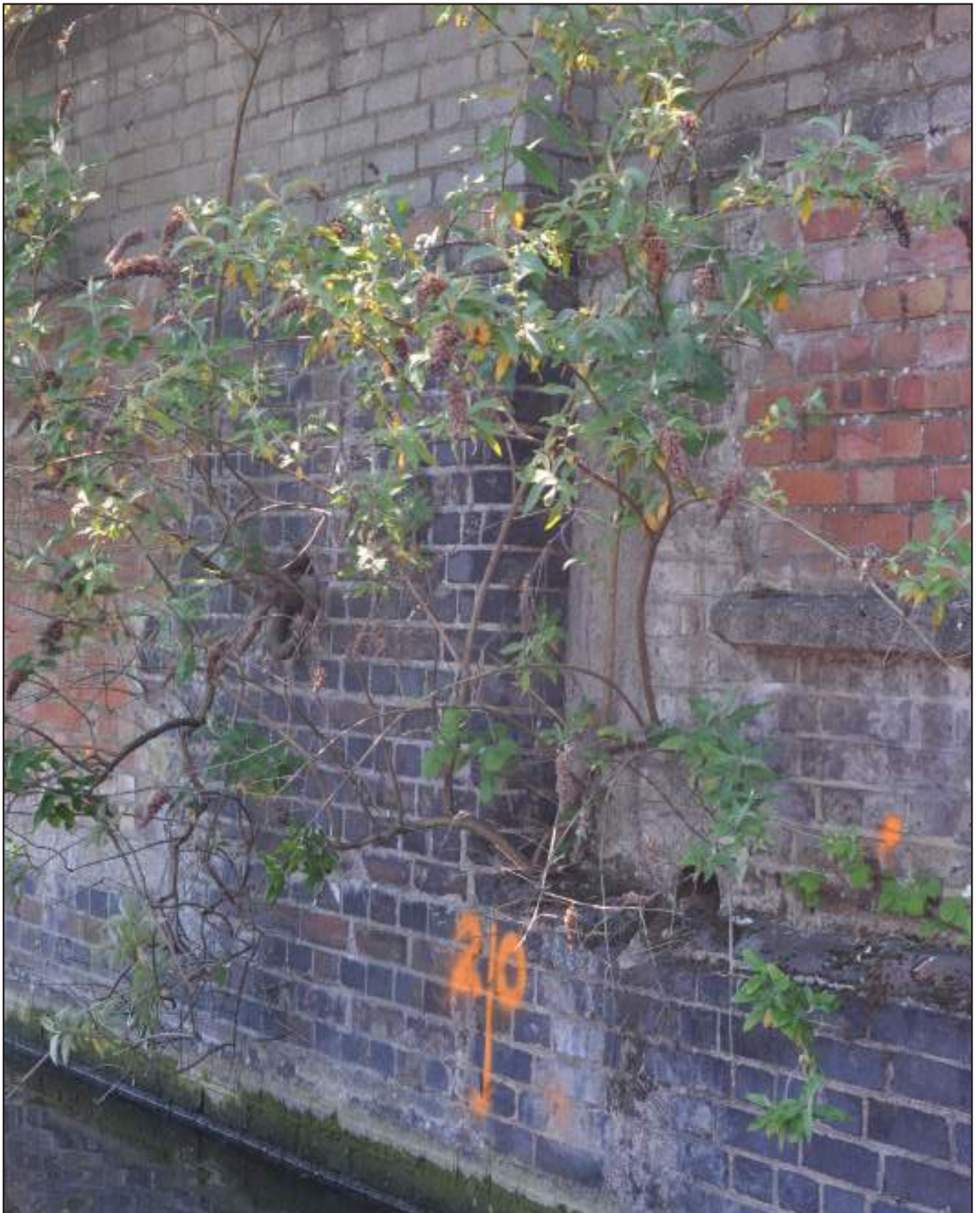
Fig.9 20m chainage - Wall alignment changes by 180mm out towards canal - blue brick
