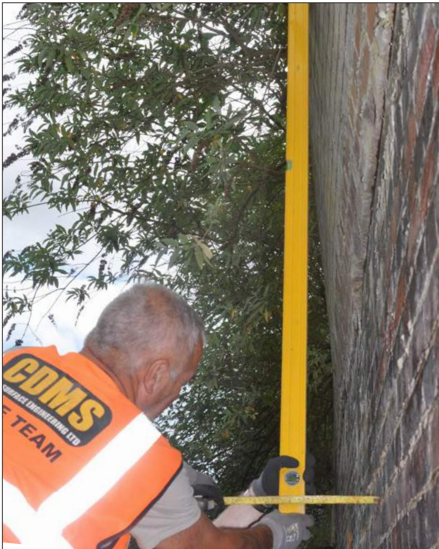
Fig.14 25.7m chainage 2 x capping / coping stones in position x 21 courses from underside to W/L dangerous misalignment to 30m chainage.
