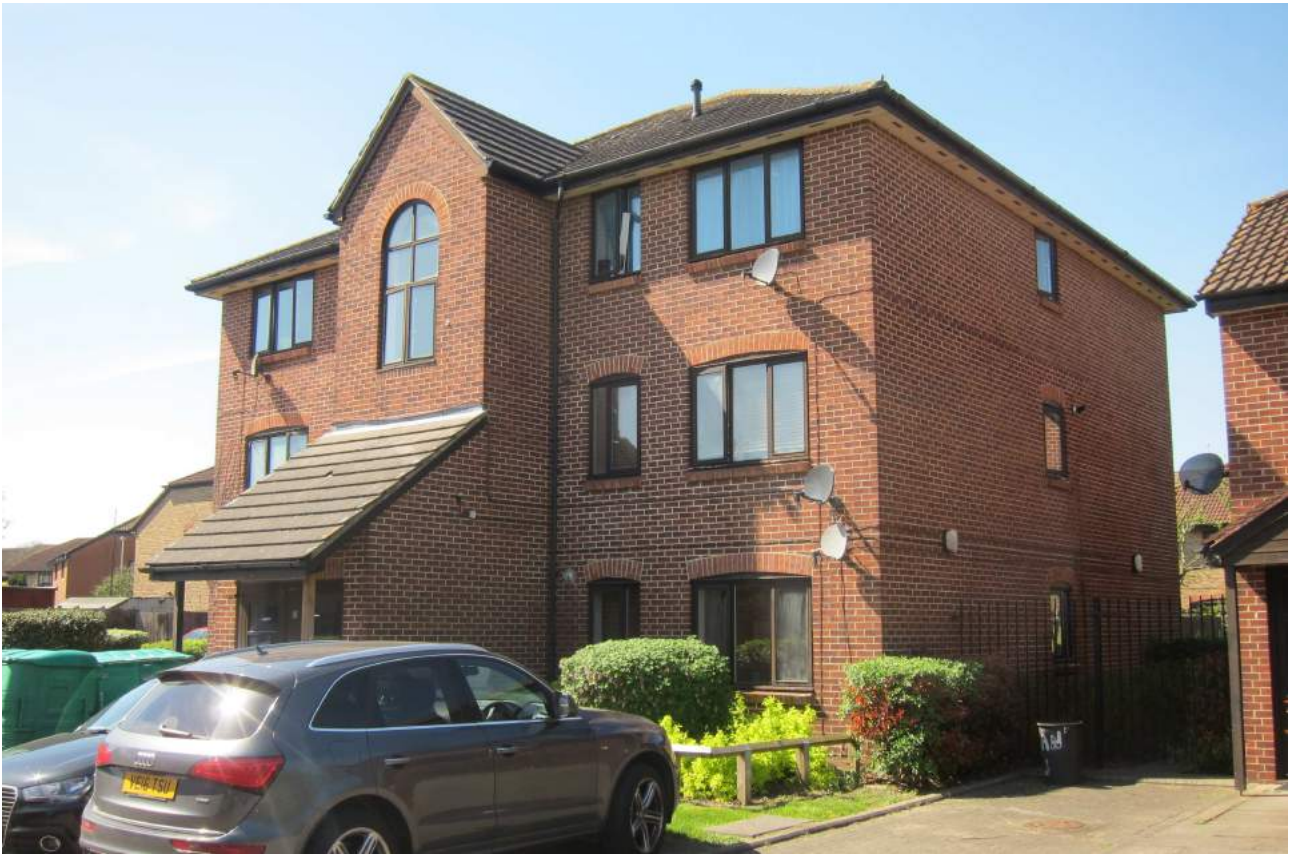
Entrance (east) and north (end) elevations
