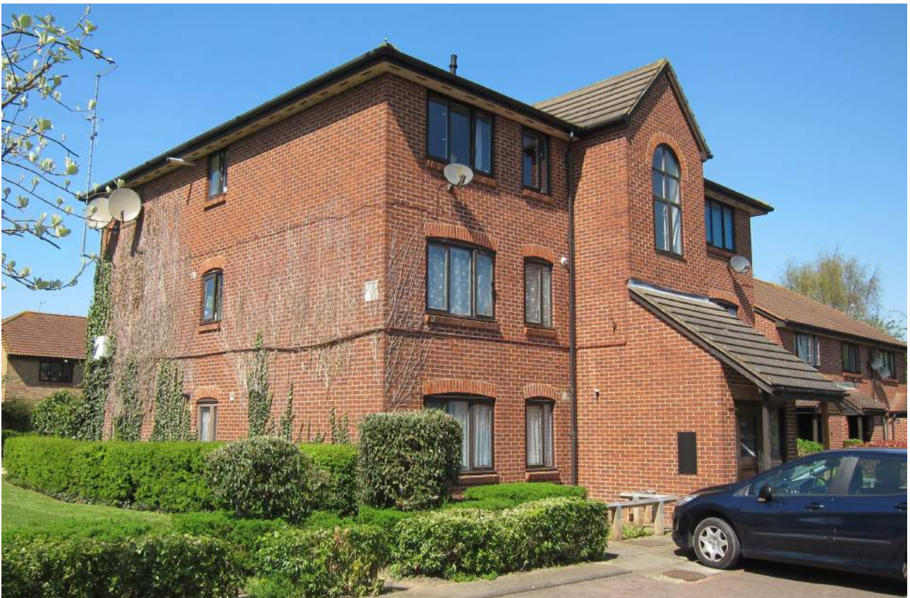
Entrance (east) and south (end) elevations
