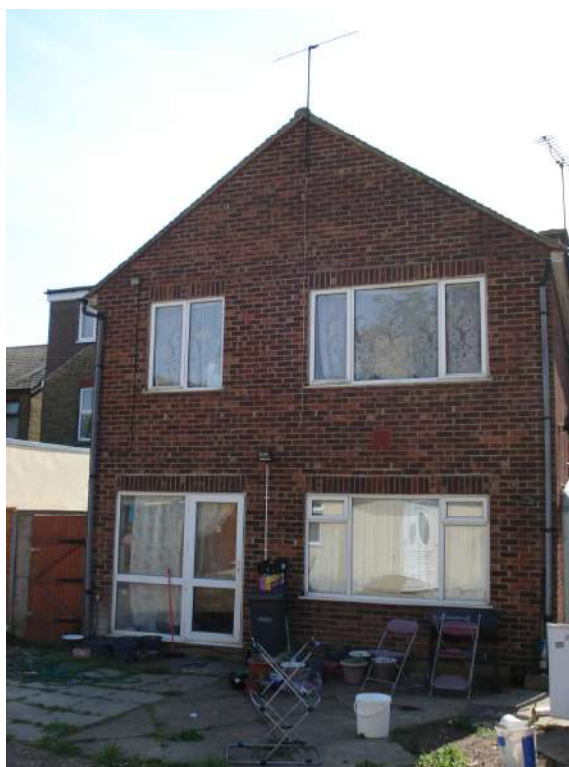
View of the rear elevation of no 226-228
