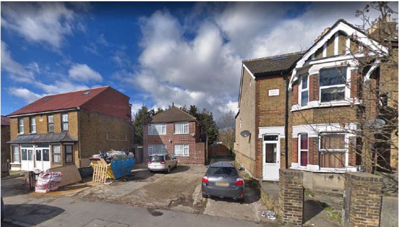
View (from left to right) of 230, 226-228 & 224 Station Road front elevations
