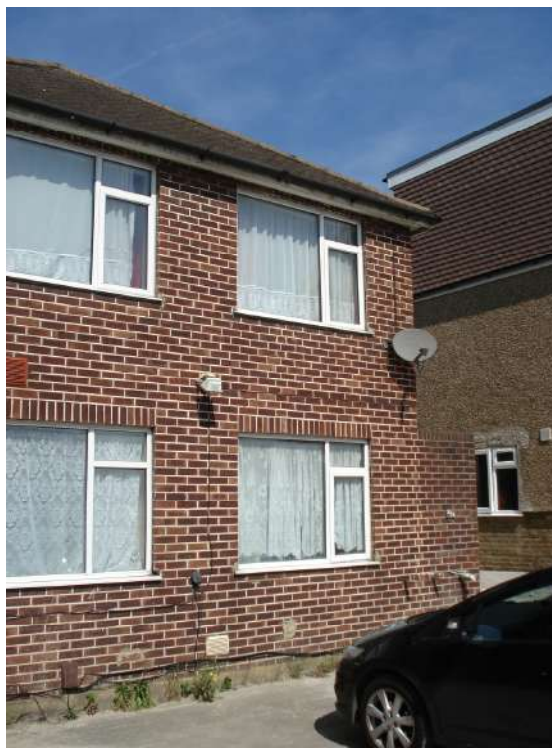
View of the front elevation of existing house from Station Road
