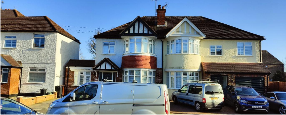
Image 1A: Nos. 78, 80 and 82 Torrington Road AS-IS: existing relationship incl. set-back between 78 and 80
