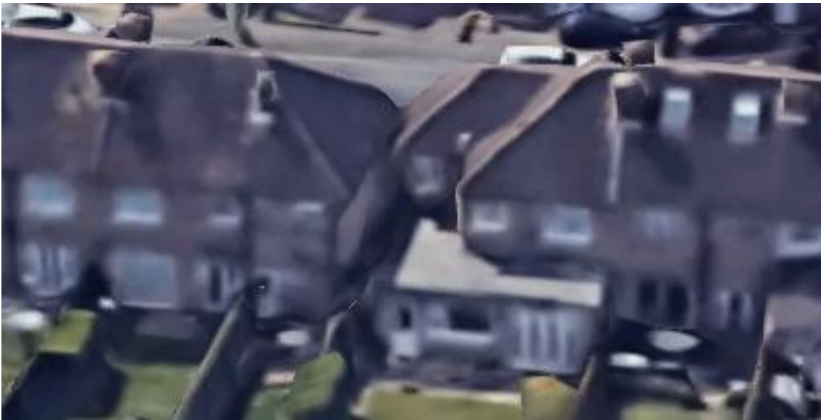
Image 5 Rear window with limited line of sight at No 7 Dartmouth Road (mitigated by additional window to the front)
