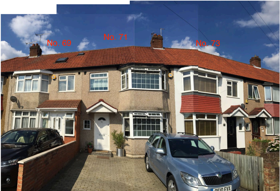
View from Lynhurst Crescent
