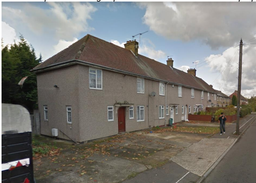
Nos. 3 to 9 West Avenue (Source: Google Street View)
