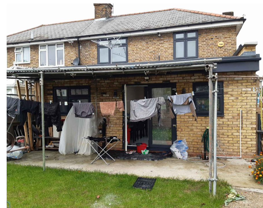
REAR OF No.18
