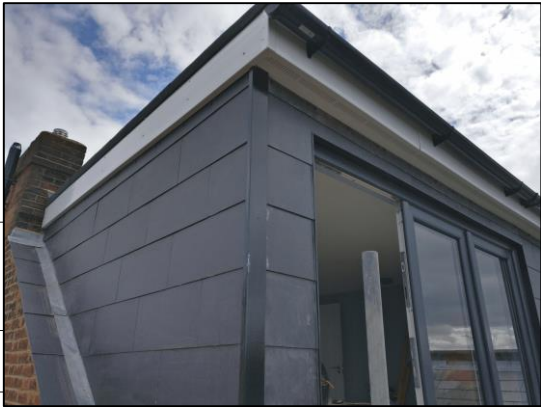
Representative example of slate to cheeks and face of dormer.
