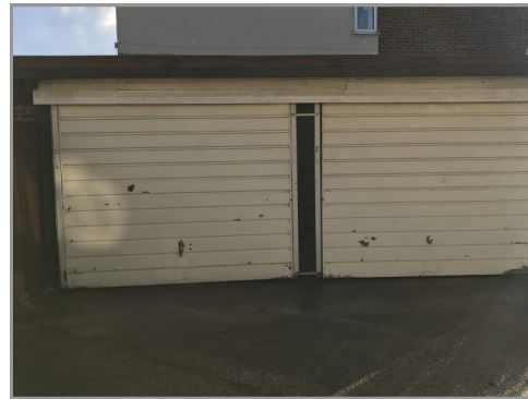
Front elevation of the existing rear garage
