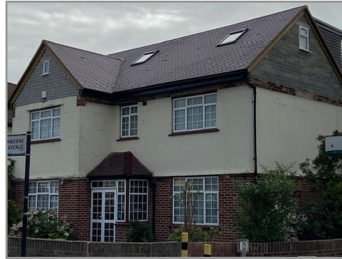
View of the side elevation of the application building from Dorchester Way
