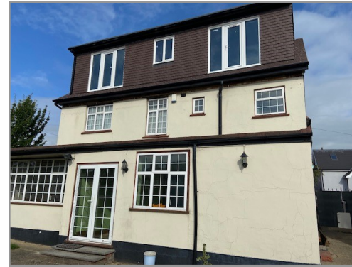
View of the application building from the rear, showing the rear dormer as existing
