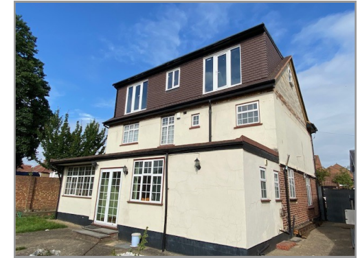
View of the application building from the rear, showing the rear dormer as existing
