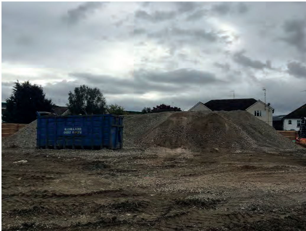
Fig 2. Stockpiled won site material, located in the southern part of the Site.
