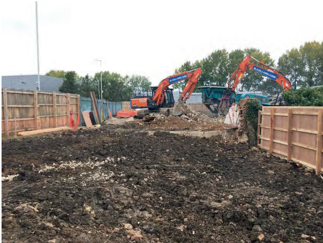
Fig 3. RCollard carrying out screening of the won site material.
