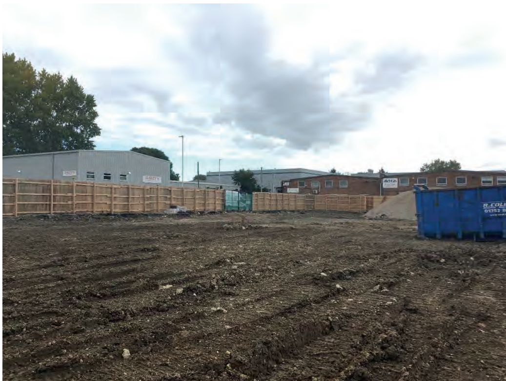
Fig 4. Northern part of the Site.
