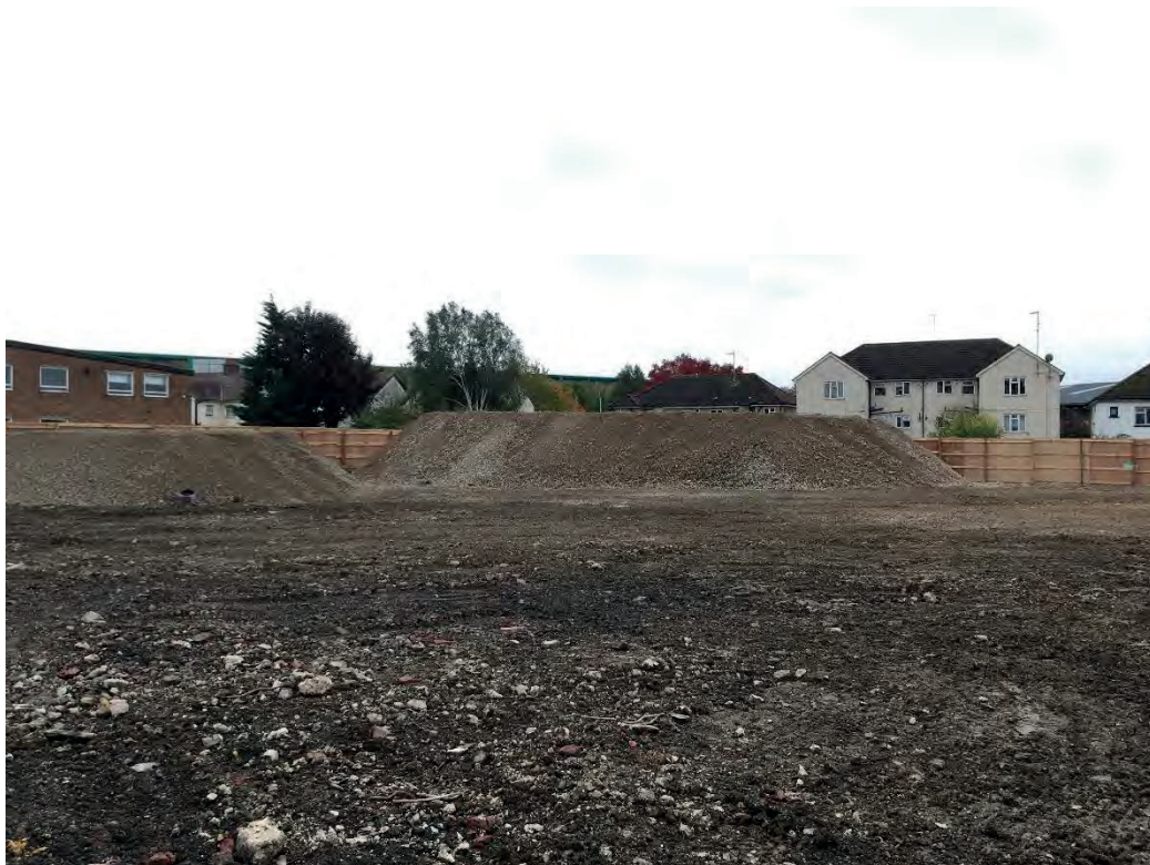
Fig 2. South eastern view of the Site with stockpiled material left on Site.
