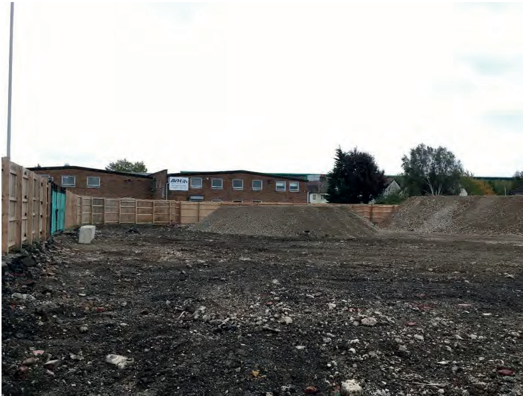
Fig 3. Eastern view of the Site with stockpiled material left on Site.
