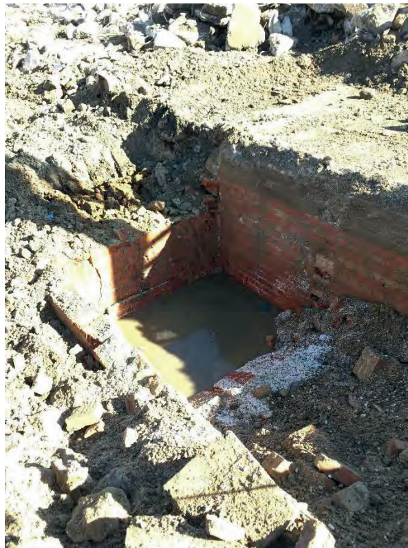
Fig 1. Excavation of DS106
