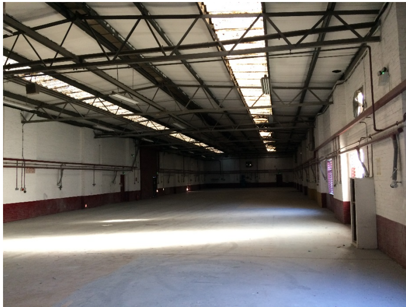
Photo 9. Internal view of building B2.
