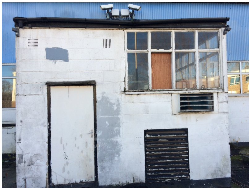
Photo 2. Northern single-storey extension of building B1 with metal louver openings.
