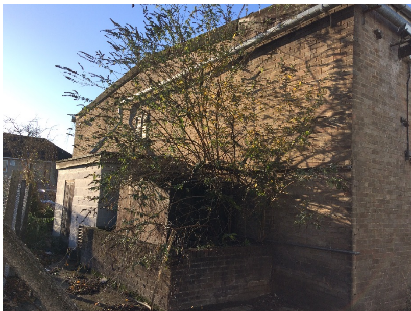
Photo 8. Eastern end of building B2.
