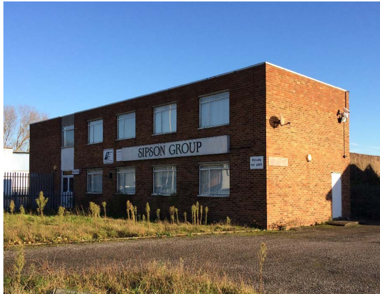
Photo 5. Building B3 from southwest, with semi-improved grassland and hardstanding in front.
