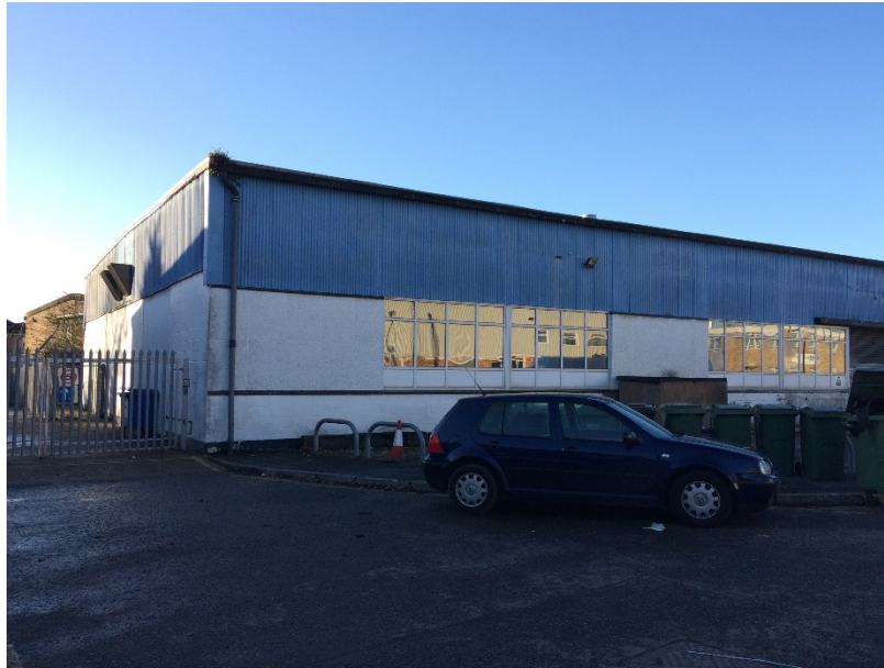
Photo 1. Building B1 from northeast, with hardstanding to north.
