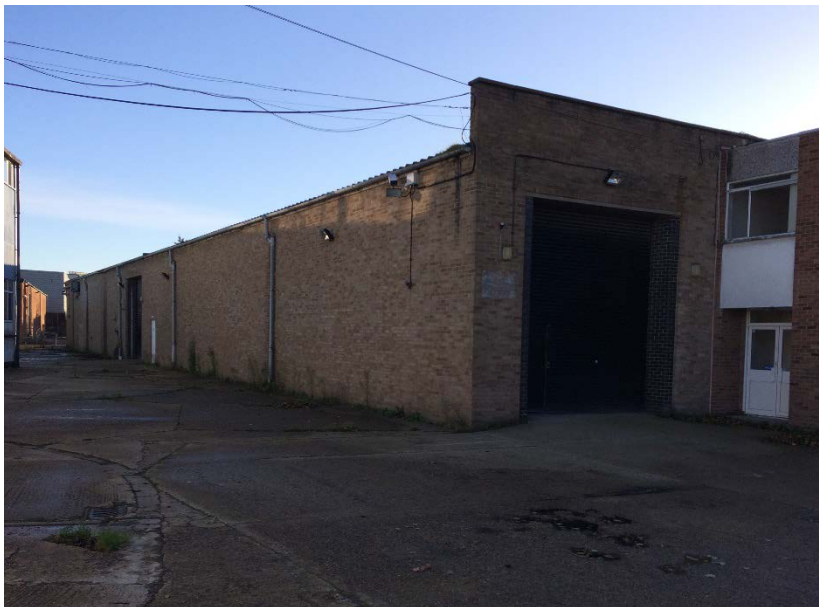
Photo 4. Building B2 from west, with hardstanding in front.
