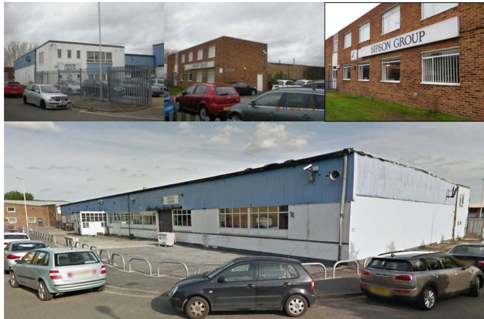
Photographs of the existing buildings on the site
