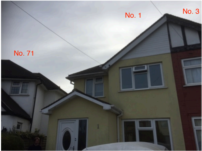
View of the front elevation of no. 1
