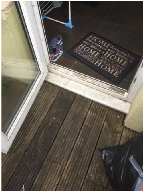
Threshold between the rear decking area and the kitchen
