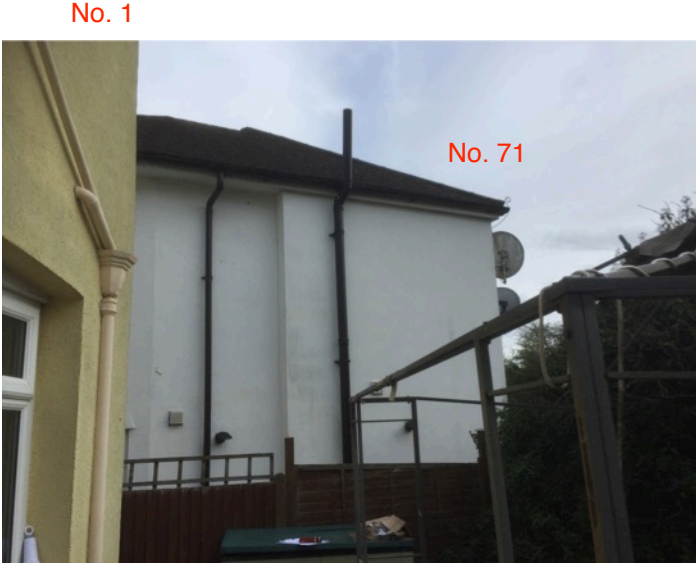
View of no. 71 from the decking area of no. 1
