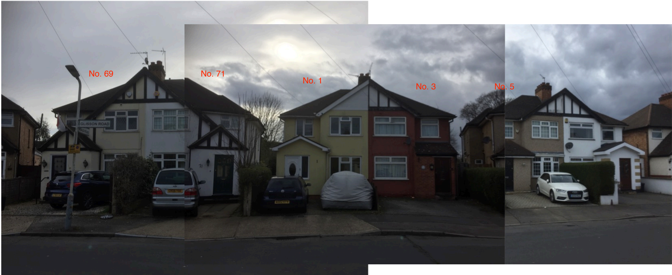
View from Glisson Road of the property
