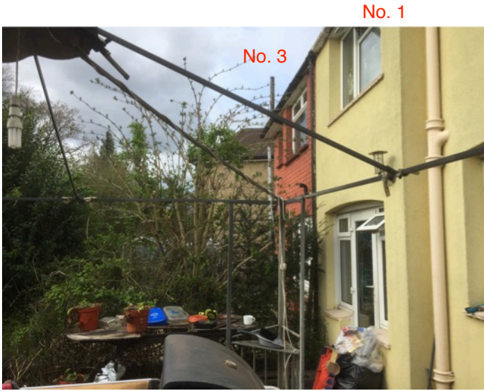
View of no. 3 from the decking area of no. 1
