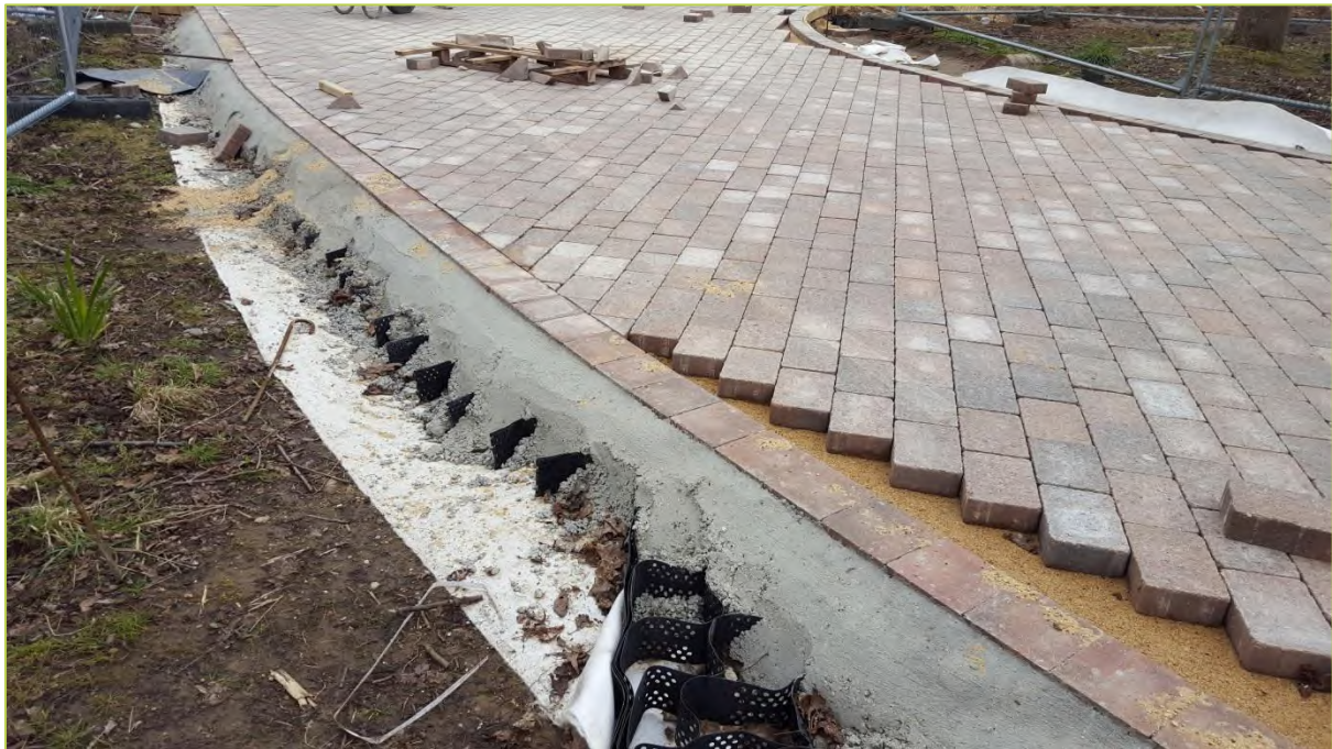
Photograph of 'Reduced-dig' 3D webbing system ground protection – 'GeoWeb' with a paver finish and kerbing installed within the sub-base cells
