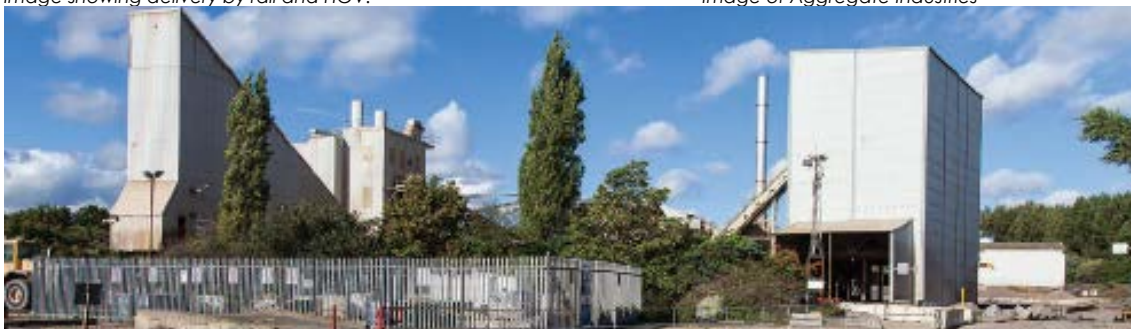
Image showing structures on site before demolition and decontamination by Aggregate Industries
