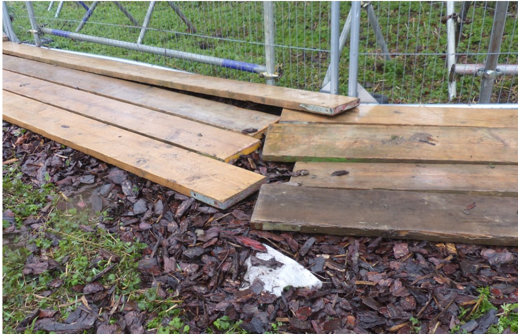
Fig 4. Scaffold boards on top of wood chips serving as ground protection. Note the geotextile layer underneath
