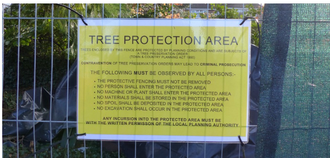
Fig 2. Signage attached to fencing reinforces the protection afforded by these barriers
