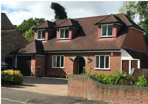
Figure 19: Catslide roofs in the locality
