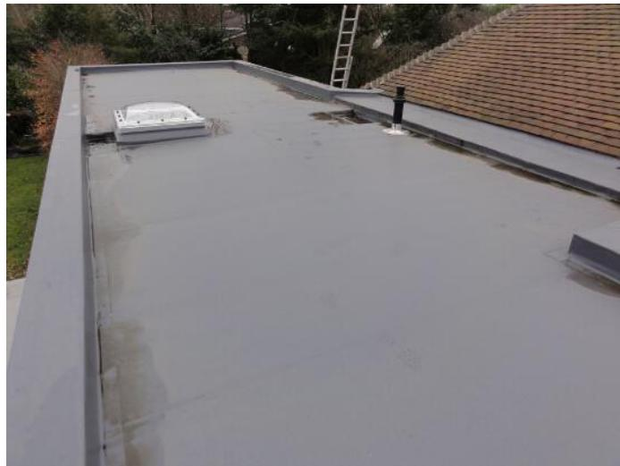
Sika-Trocal Single ply Polymeric roofing membrane
