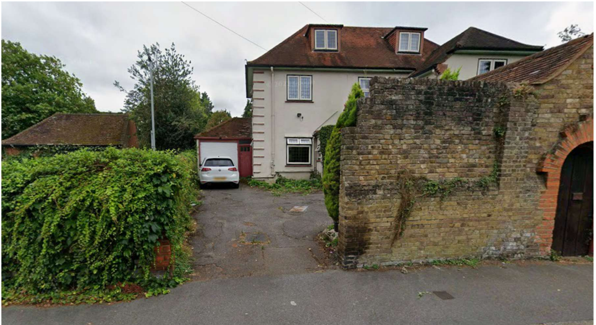
Figure 2-1: Existing Access to the Site
