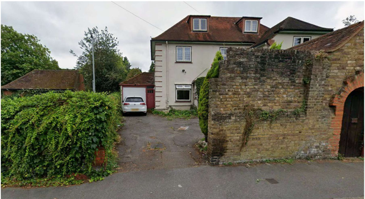
Figure 2-1: Existing Access to the Site
