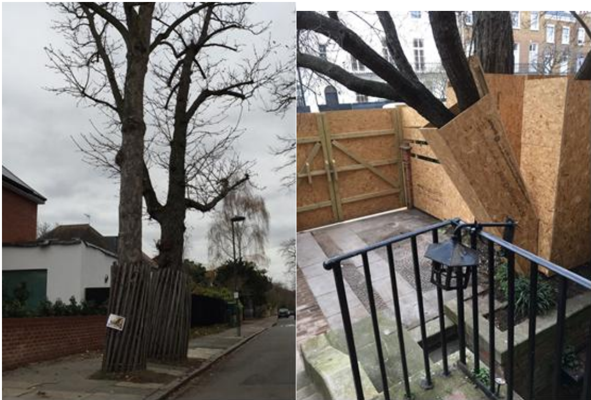
Photo 2: Trees protected by hessian & chestnut pale fencing / limbs protected by wooden boxing
