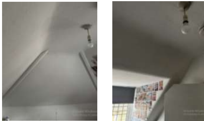
Figure 3 Photographs of loft conversion.
